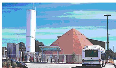
(Left) The Hydrogen Fueling Station at the city of Chicago. Shown in the photo is Chicago's Fuel Cell Public Transit Vehicle. The solar panel, next to the hydrogen storage tank (vertical column), is used to supply power needed to decompose water into hydrogen and oxygen. Hence, from the production of hydrogen gas to its usage in the fuel cell vehicles, it is 100% environmentally friendly.
